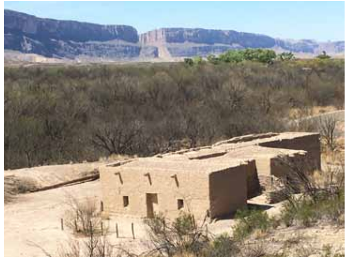
Adobe home built in 1901 by Cipriano Hernandez and used as the first store in Castolon, with a view of Santa Elena Canyon.
